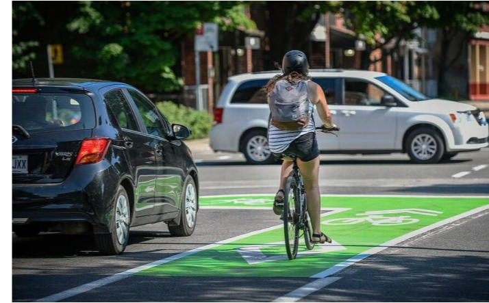
Fig.71. Example of a bicycle path at intersections, Ottawa, Canada Source : Ville d'Ottawa
