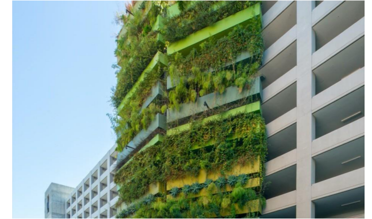
Fig.117. Green facade, Los Angeles, US
