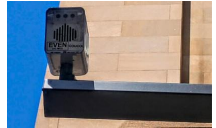
Fig.127. Auditory signal device at intersections Source : Ville de Montréal
