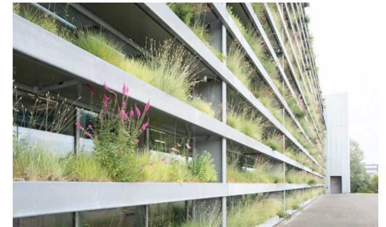
Fig.119. Green sunbreaker on multi-storey parking lot, Switzerland
