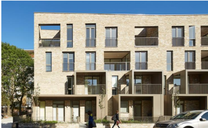
Fig.97. Ely Court quadruplex, London, UK Source : SKE Portico
