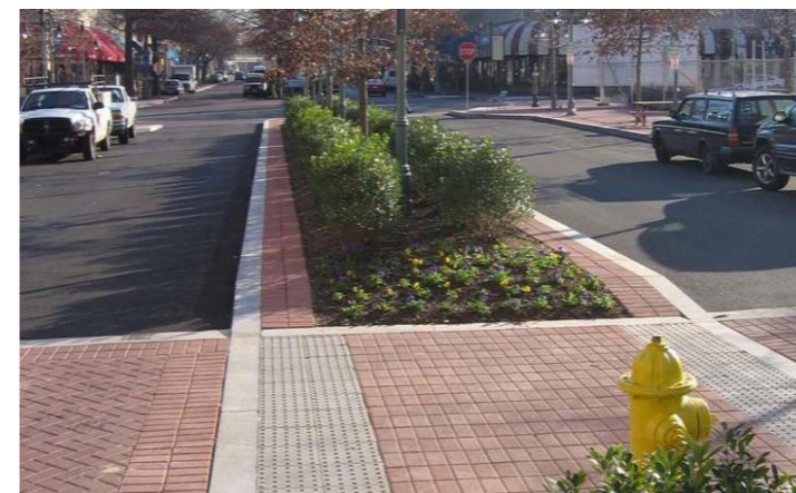
Fig.77. Pedestrian crossing with a central island, Arlington, Virginia, US Source : NACTO
