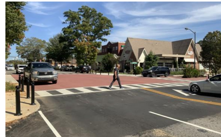
Fig.73. Elevated intersection, Matthew, North Carolina, US Source : NACTO
