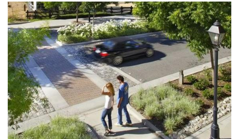
Fig.74. Elevated pedestrian crossing, Santa Monica, US Source : RRM Design Group
