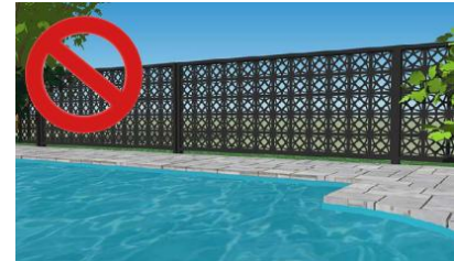
Figure 7 Example of a fence that could facilitate climbing
